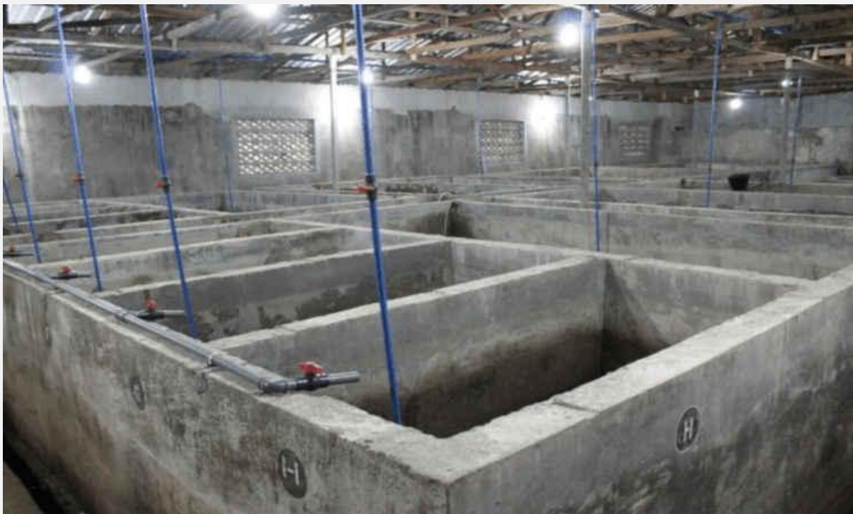
Picture 4.4: Concrete tanks built in an enclosed housing space to house fish; Source – Everlush.ng
