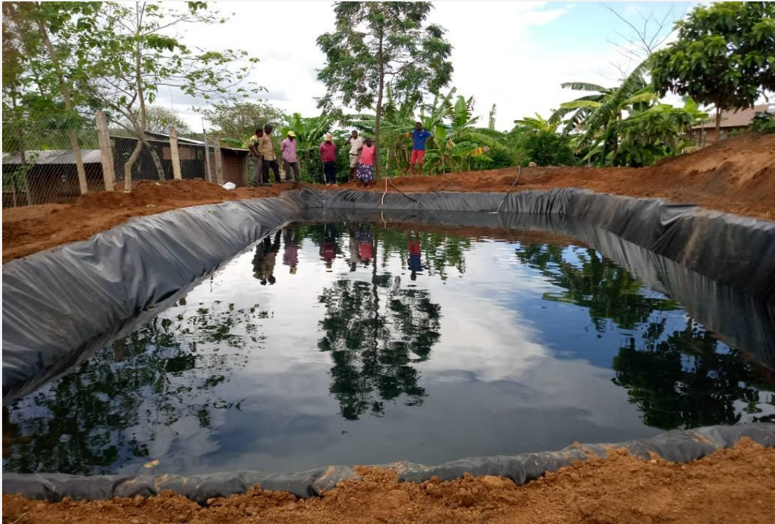
Picture 4.6: Tarpaulin Pond set-up to house fish with tarpaulin material placed in a dug-out earthen space; Source – Everlush.ng
