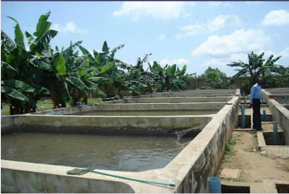
Picture 4.3: Concrete tanks constructed to house fish; Source – Business Compiler
