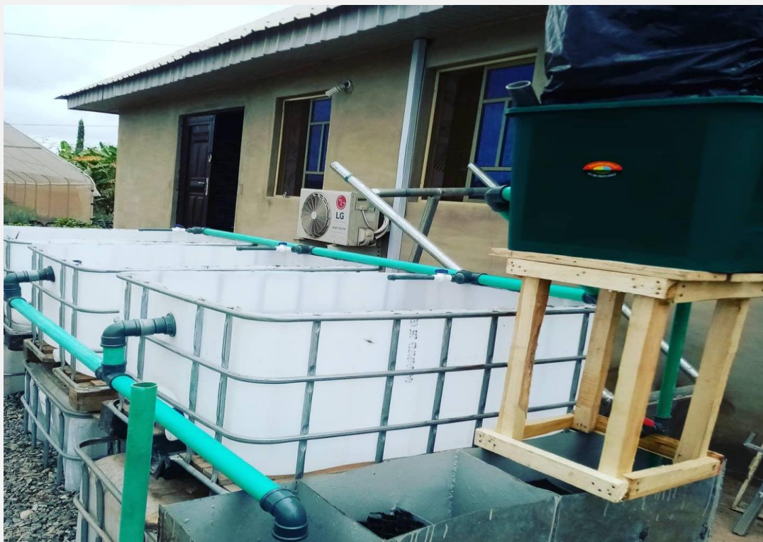
Picture 4.7: Small-scale Backyard RAS Fish Pond set-up; (Source – Hydroponics Nigeria )
